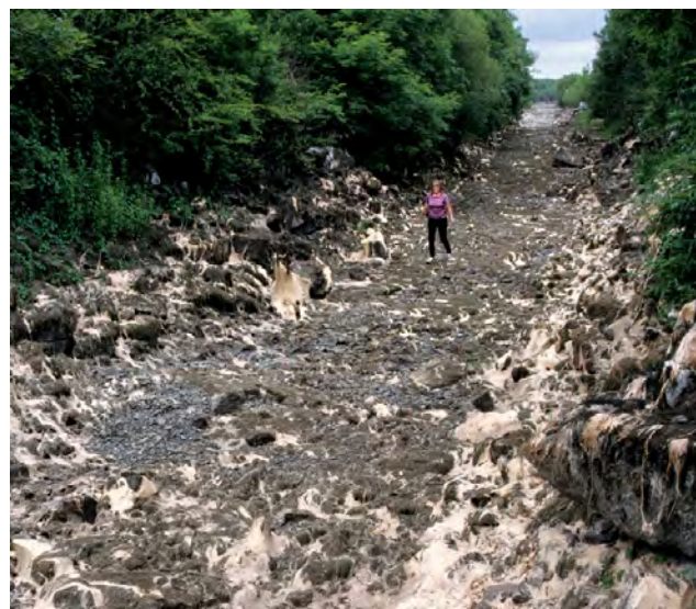
Fig. 5. Karst hazard. The Cong Canal in western Ireland that does not hold water because it was built on karst limestone.
