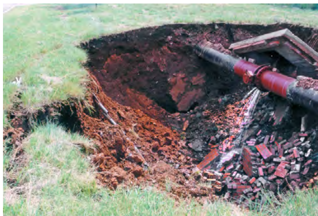
Fig. 23. A small, new subsidence sinkhole in soil-covered dolomite karst in South Africa, clearly induced by the leakage from the water pipeline that is now exposed (photograph by courtesy of the late Fred Bell).
