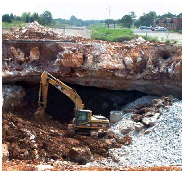
Fig. 19. The collapse sinkhole that destroyed Dishman Lane in Kentucky, with an initial failure where ground collapsed into the wide cave less than 5 m below the surface. This image was taken when collapse debris had been removed prior to installing a stable fill. The thin cave roof is exposed in profile, with some of the deep soil-filled fissures and miniature buried sinkholes visible above the arm of the backhoe (photograph by courtesy of Hilary Lambert).
