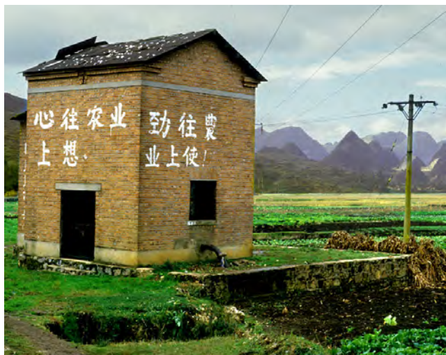
Fig. 11. One of the pump-houses over wells into the limestone of the Shuicheng basin in China. The small new sinkhole just metres from it has been caused by water and soil descending into the cone of depression, aided by leakage from the broken pipe where it emerges from the building.
